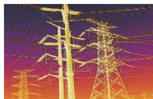
Electric Routine Inspection
