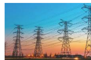
Electric Device Routine Inspection
