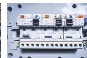
Electric Routine Inspection
