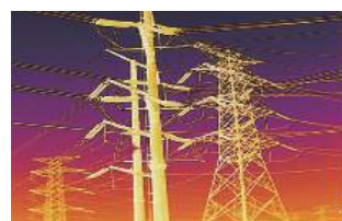
Electric Routine Inspection
