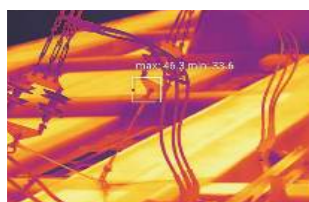
Electric Routine Inspection
